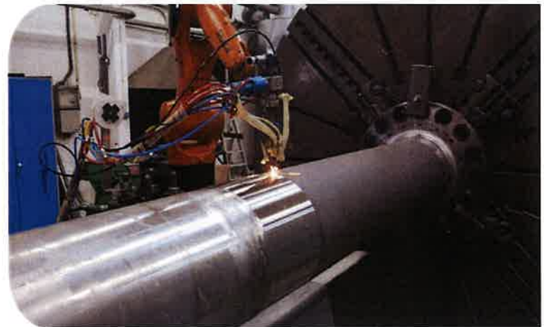
Laser cladding of seal surface
